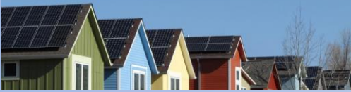
City of Boulder: emergency center, shelter, wildfire center, wastewater treatment, public housing
